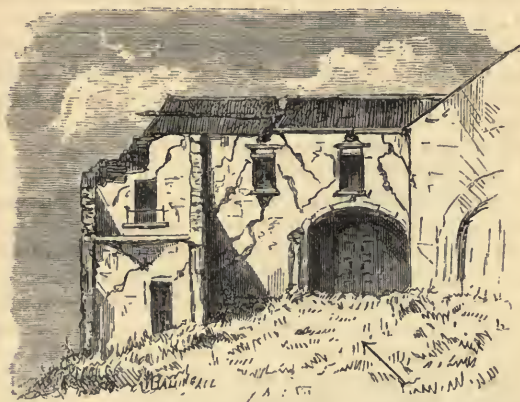
FIG. 38.—House rent by earthquake (Mallet). The arrow shows the direction from which the earthquake-wave must have reached the surface.
